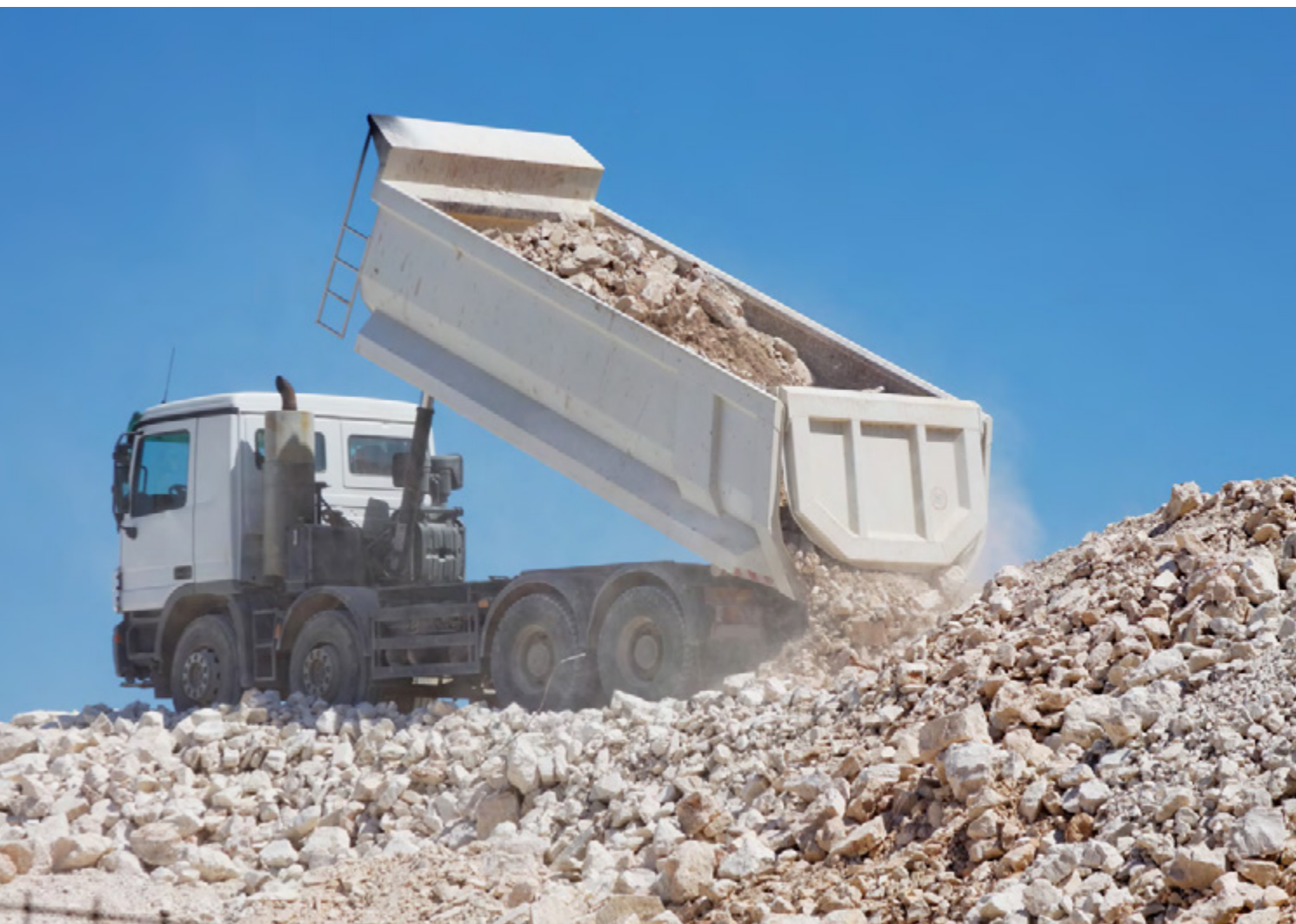
Tipper truck unloading crushed rock
